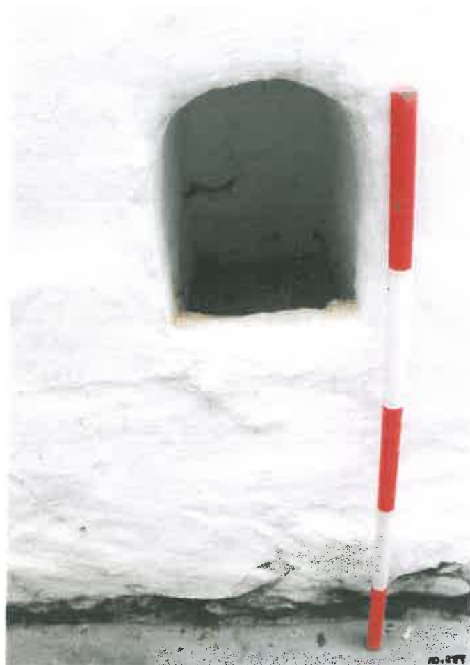
6.2 One of the lower hen-nests with its rounded humps to prevent eggs from rolling out.
