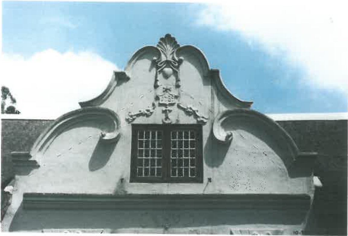
28. When one looks carefully at the front gable, the old lines where the tin roof clipped the gable, is obvious.
