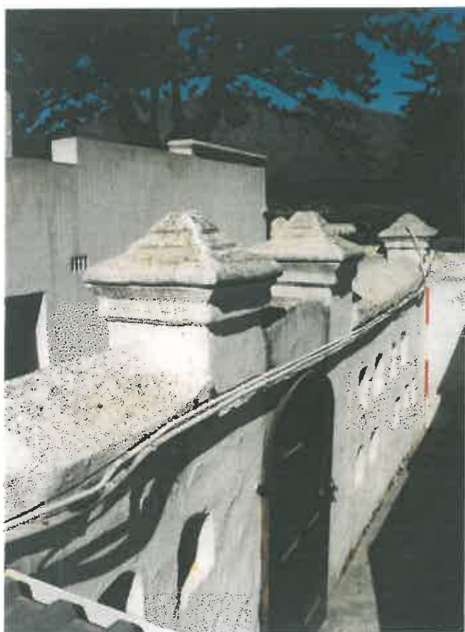
80. The door to the entrance of the fowl-run date to the time of Palmes, and should be fitted on the other side of the wall (scale 2m)(looking E).
