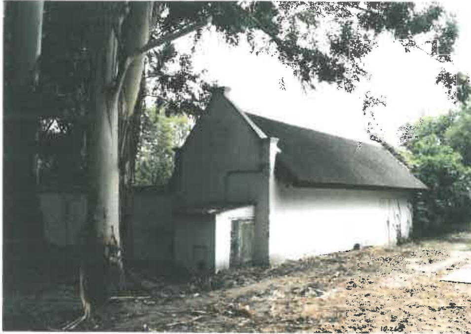
20. The bathhouse of 1952 with its cottage-styled thatch.
