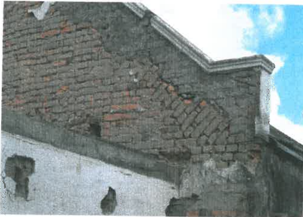
122. Close-up of the oblique brickwork (northern end)(J. Malherbe).
