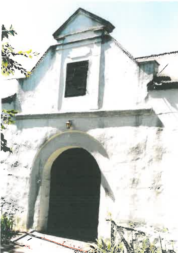
8. The existing gable was presumably also clipped in the late 1800s and partially reconstructed >1950.
