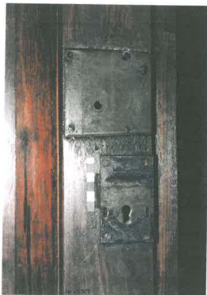
33. The old lock with its handmade nails is above the later 19 th century doorlock with its screws (scale 5cm).
