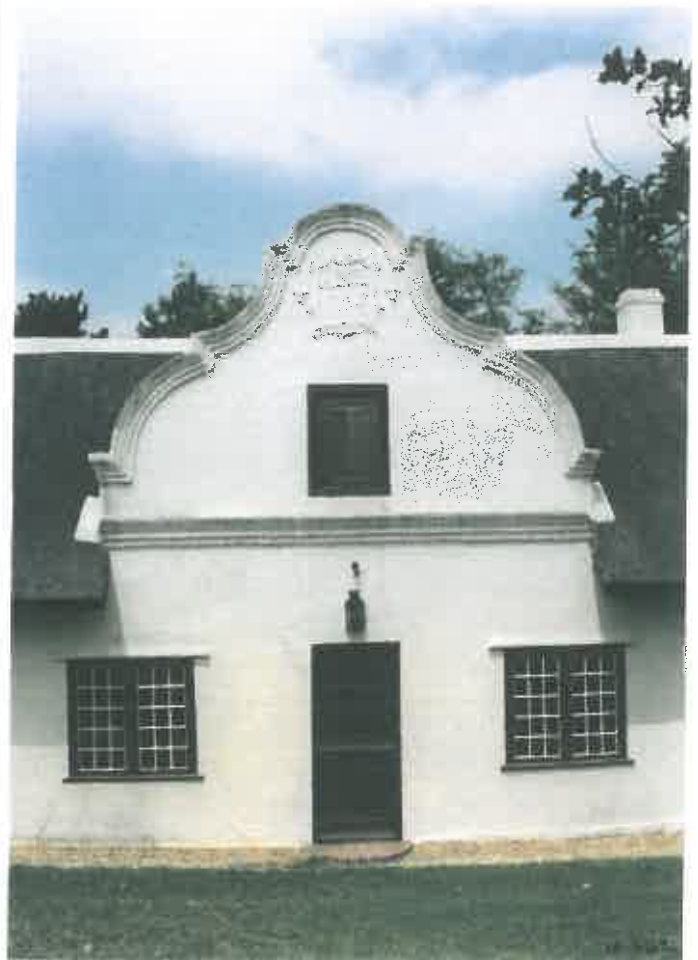
97. Afterwards a new dormer shutter was put in place.
