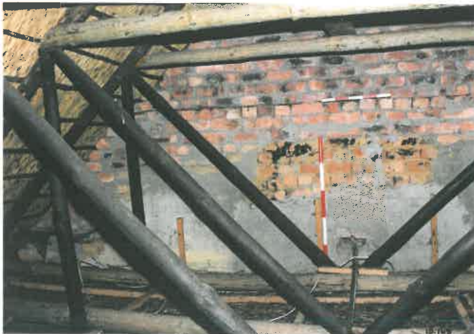
108. In the loft, wall E2 show signs of black soot on the brick and mortar, indicating a chimney at one time (scales 1m & 50cm)(looking E).
