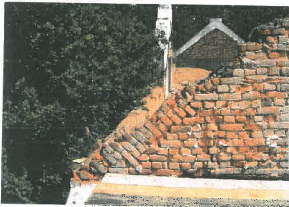
123. Close-up of the oblique brickwork (southern end)(J. Malherbe).
