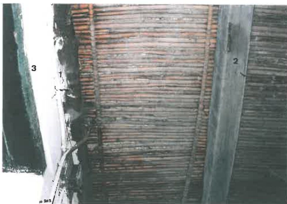
124. A view of the 19 th century reedloft ( brandsolder ) with the poplar beam (1), the old beam (2) and the 18 th century lintel (3).
