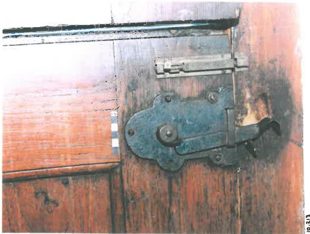
39. On the lower half of the front door is the (presumably) original coil-spring-loaded latch.
