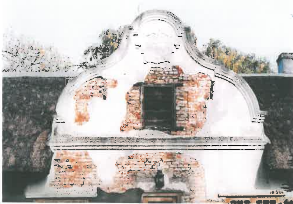
95. During the 1979 renovations, the old brickwork below the plaster revealed that a double casement once adorned the gable.
