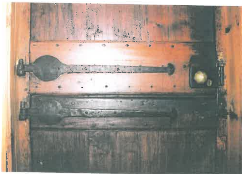
66. Note the geometric scale designed for spacing the nails evenly.
