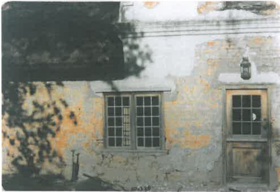
98. Immediately east of the double casement (in an old position) was an old door blocked up in brownish bricks (courtesy GB).
