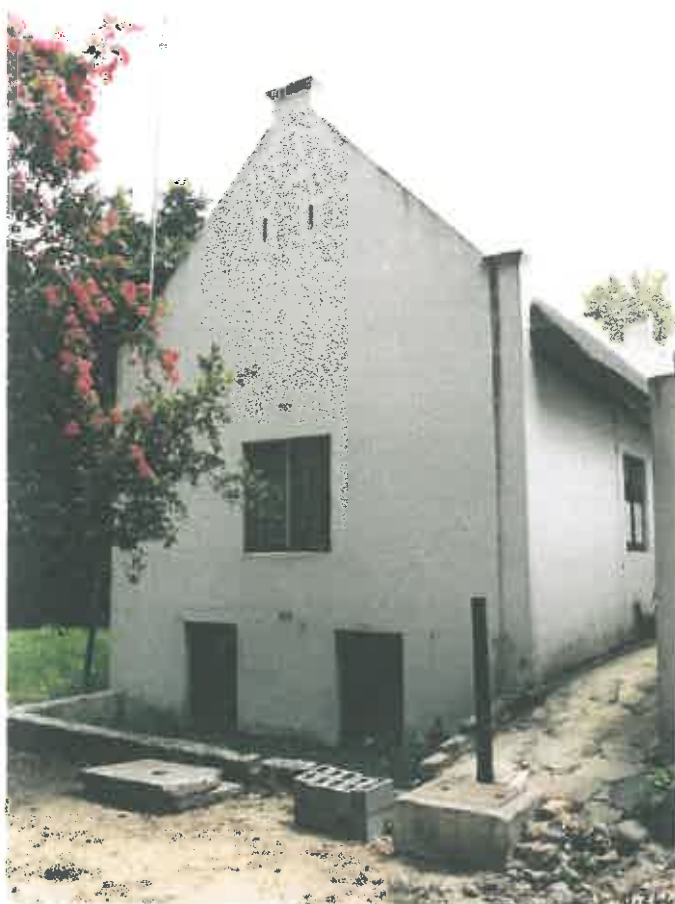
85. Two small doors leads to a basement cellar below the quarters of the staff.
