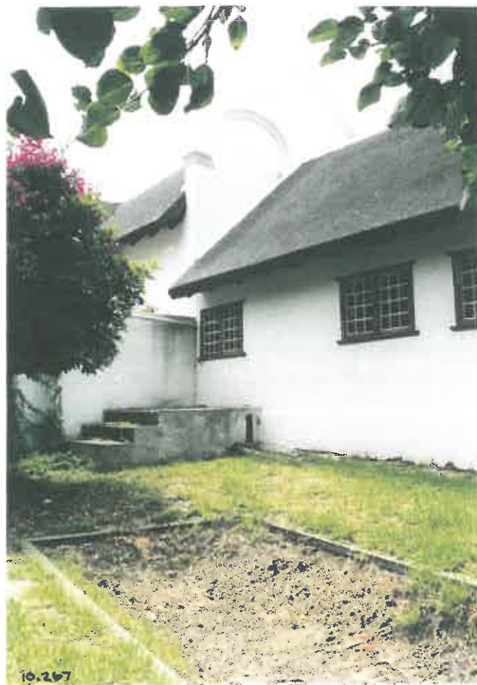
88. According to GB, these steps originally gave access to the kitchen of Palmes (>1950), via the old kitchen door. Prior to this, the door was situated in the visible end-gable wall.
