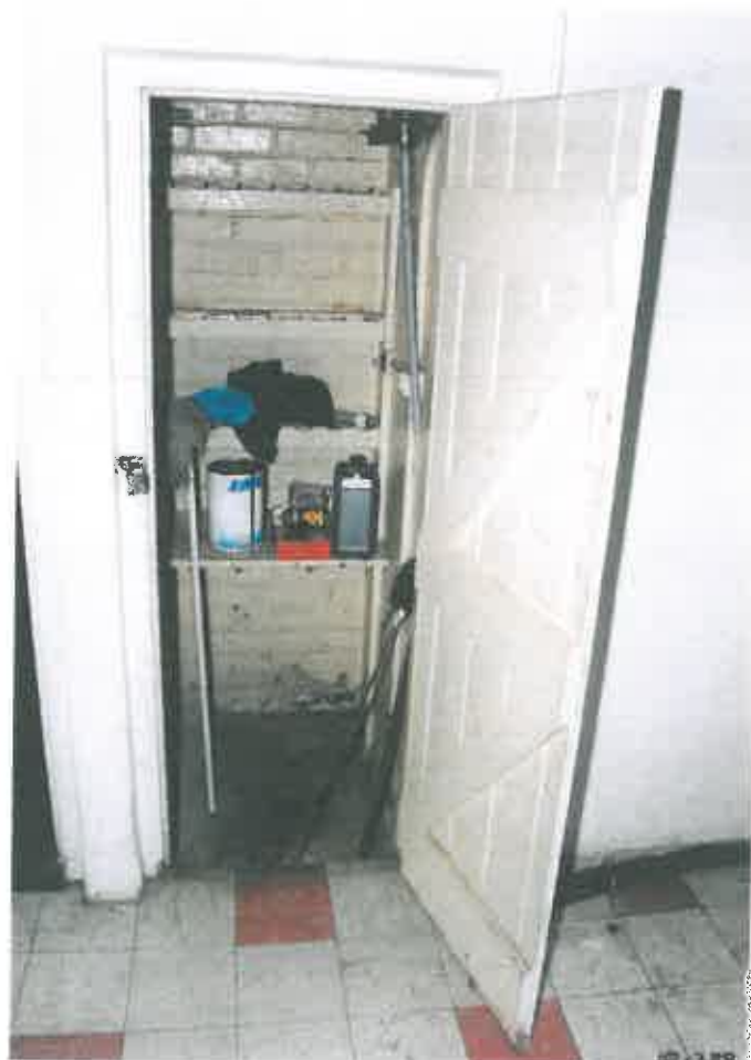
86. This cupboard now encloses a number of steps which led to a storage basement, now filled with riverstones (GB via Kinahan).
