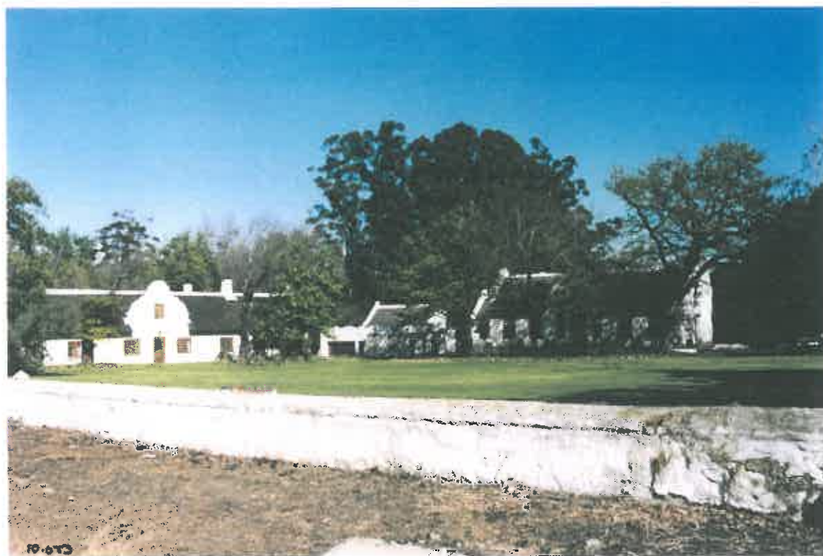
141. The crooked boundary wall has been rebuilt with riverstones for much of its length.
