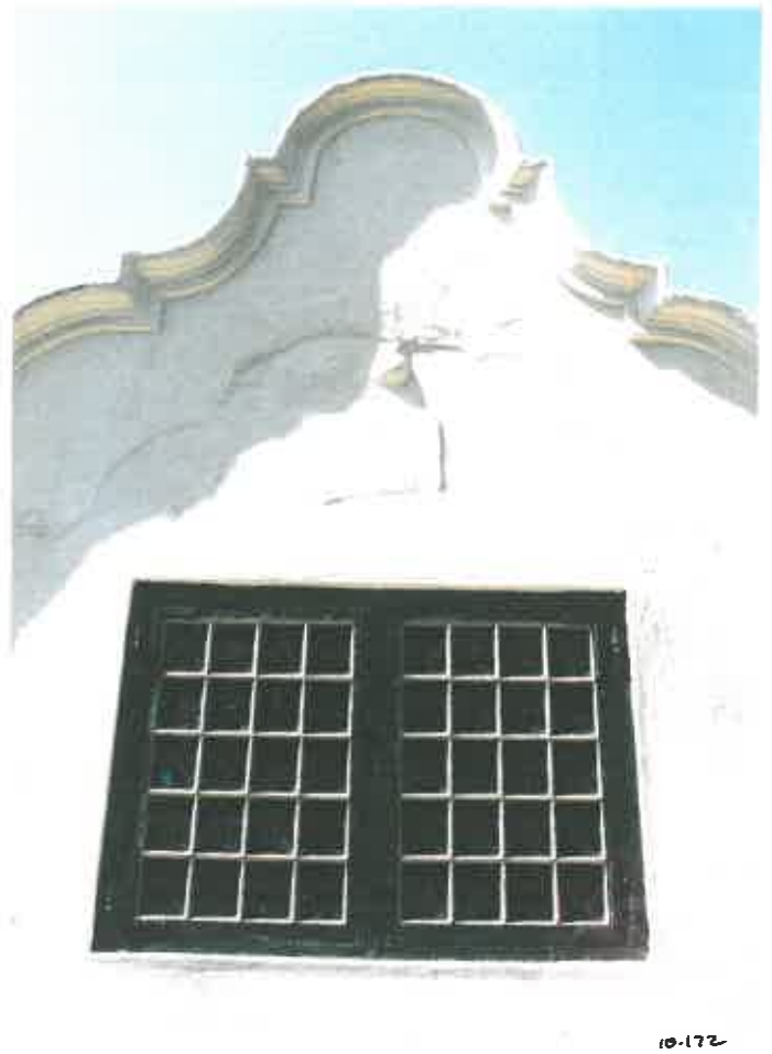
118. The casement is fully restored with its new window panes.
