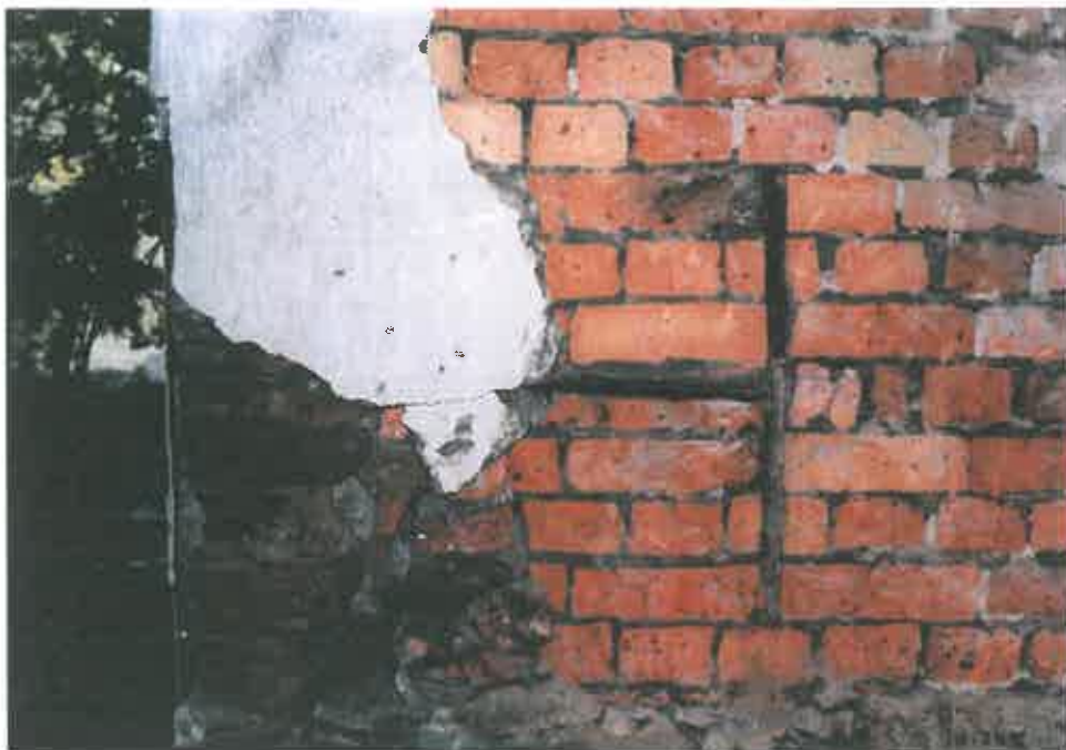
103. In the eastern end-gable the rear portion of the wall was stabilised by letting two iron ties into the early 18 th century brickwork.
