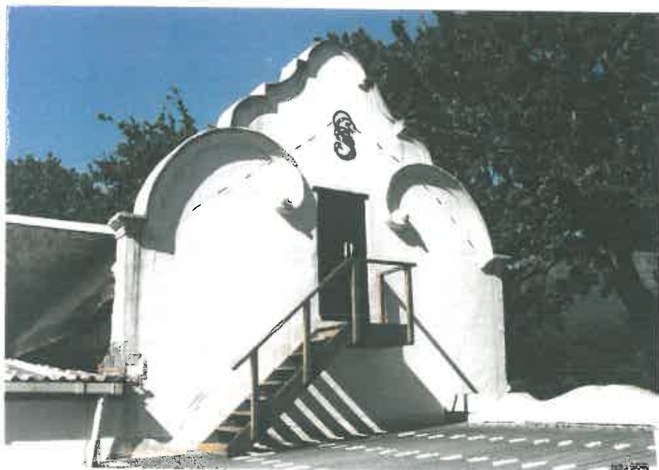
19. The clipped endgables were reconstructed after 1952 by Palmes, who used the architect J.B. Collins. Note the old lines of the corrugated roof (looking N).
