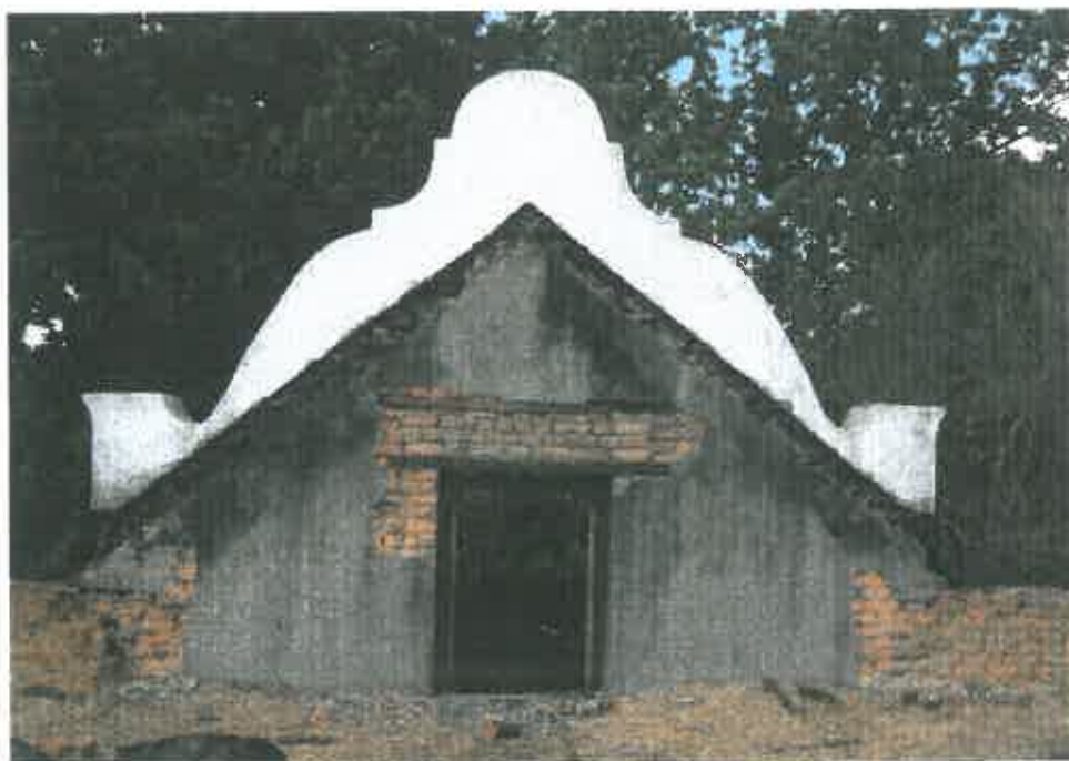
115. In 2001, when the corrugated roof was taken off, the later, white “cemented” gable was clearly outlined (looking S)(Courtesy J. Malherbe).
