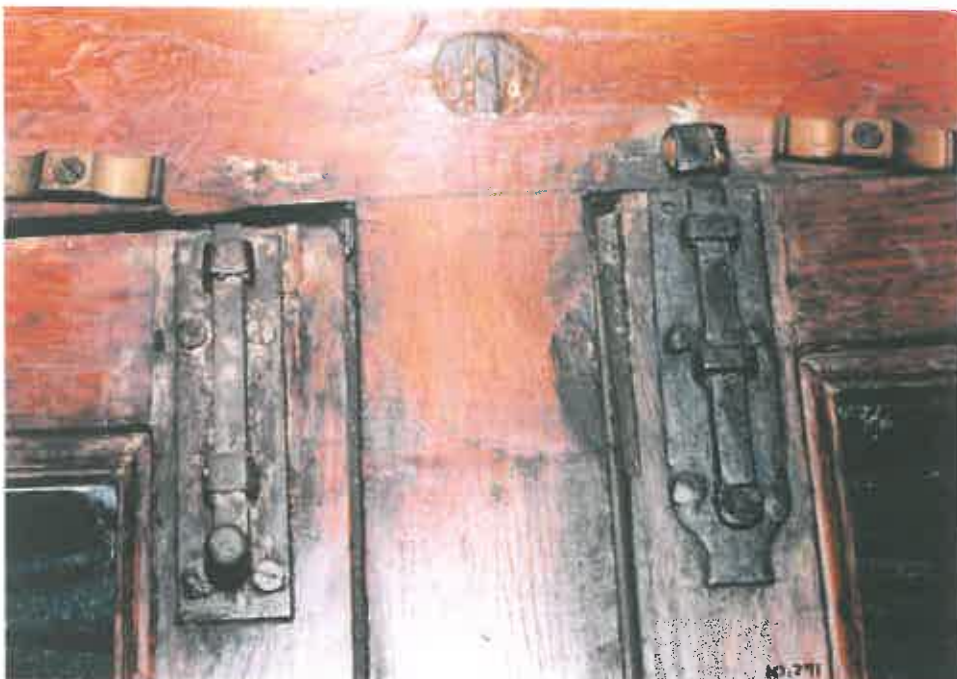
53. On the interior of the rear casements are these sliding bolts (upper portion). The left one is a replacement (19 th century).
