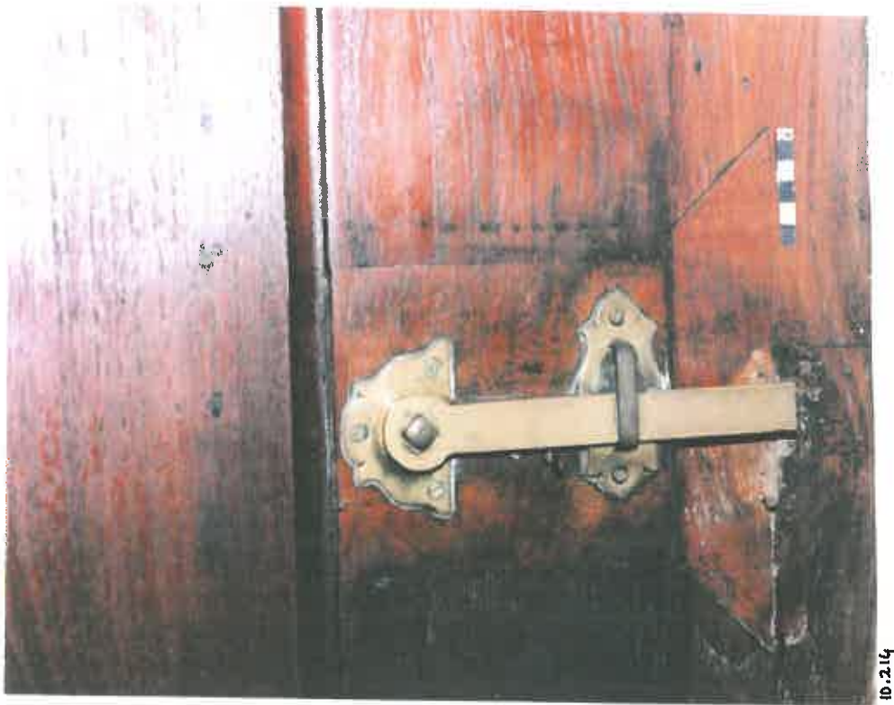
38. The solid brass latch (>1950), imposed where the old front door lock was situated (note the replacement wood)(scale 5cm)(looking E).
