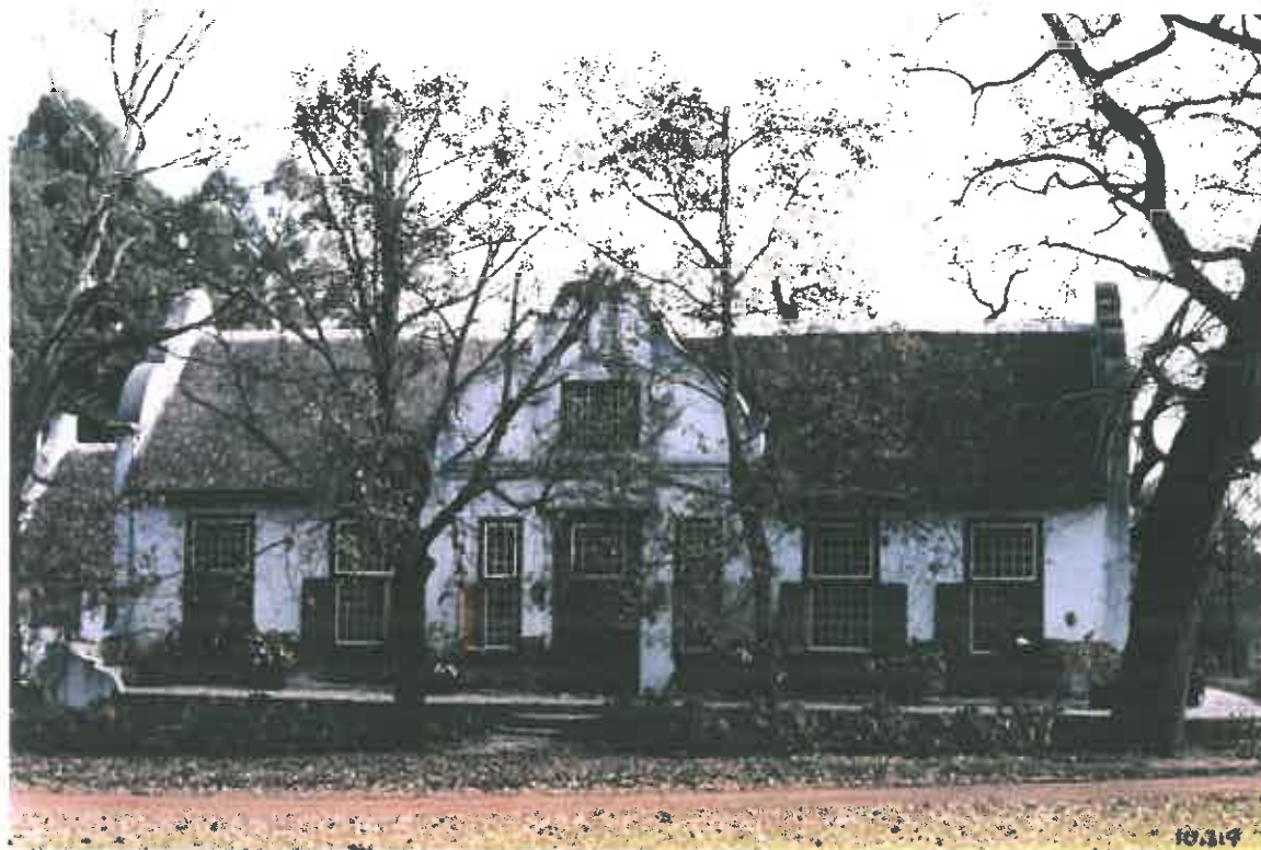
26. A view of the façade during renovations. Note on the far right a small patch of remnant plaster.
