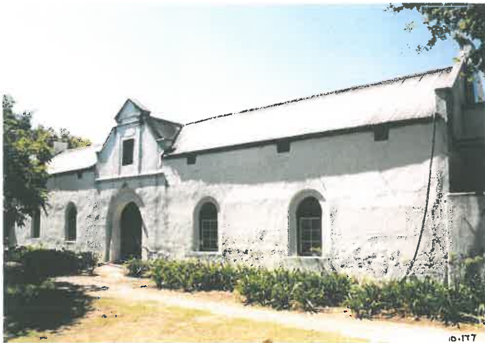
126. A view of the c.1820 façade of the wine-cellar, showing its old plasterwork, built-up eaves, ventilation grids and corrugated roof.
