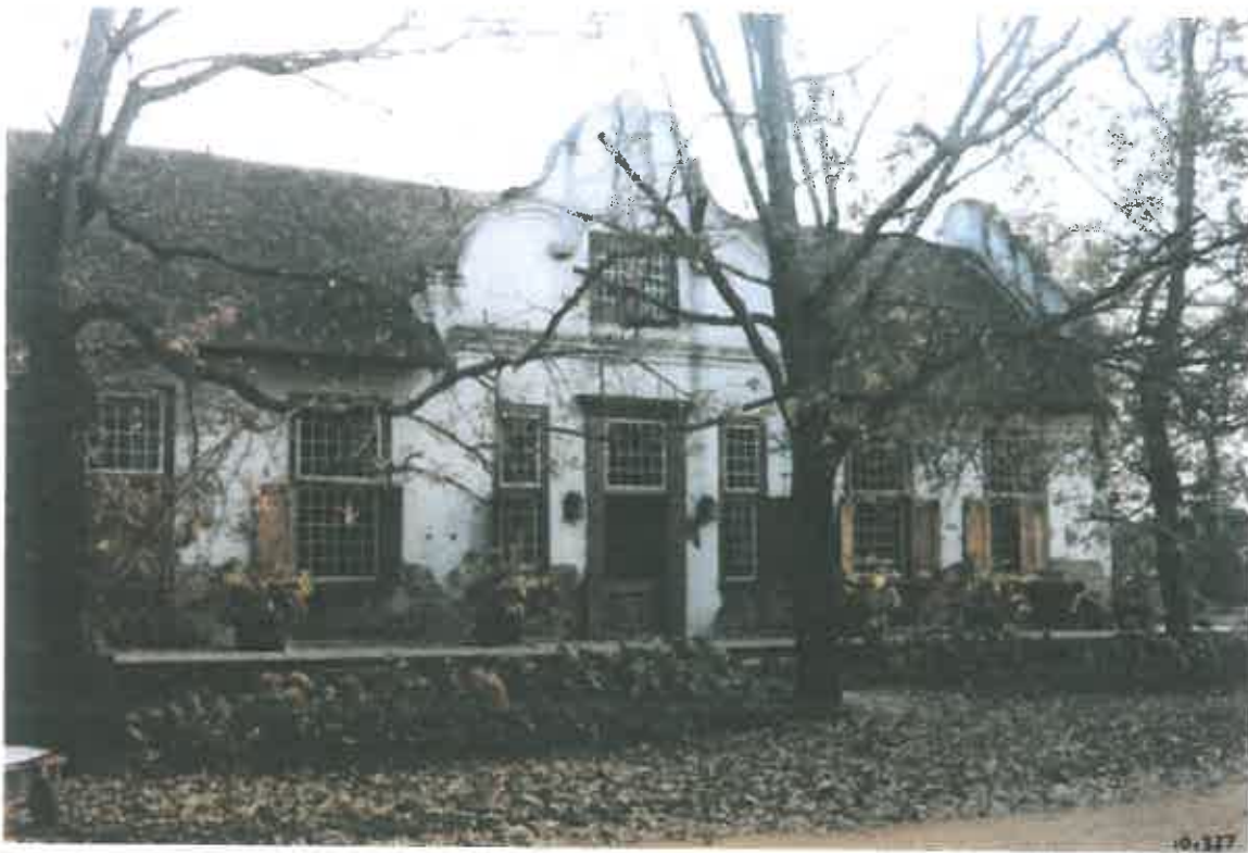
23. In June 1979 the lower part of the façade wall above the stoep was stripped (courtesy GB).
