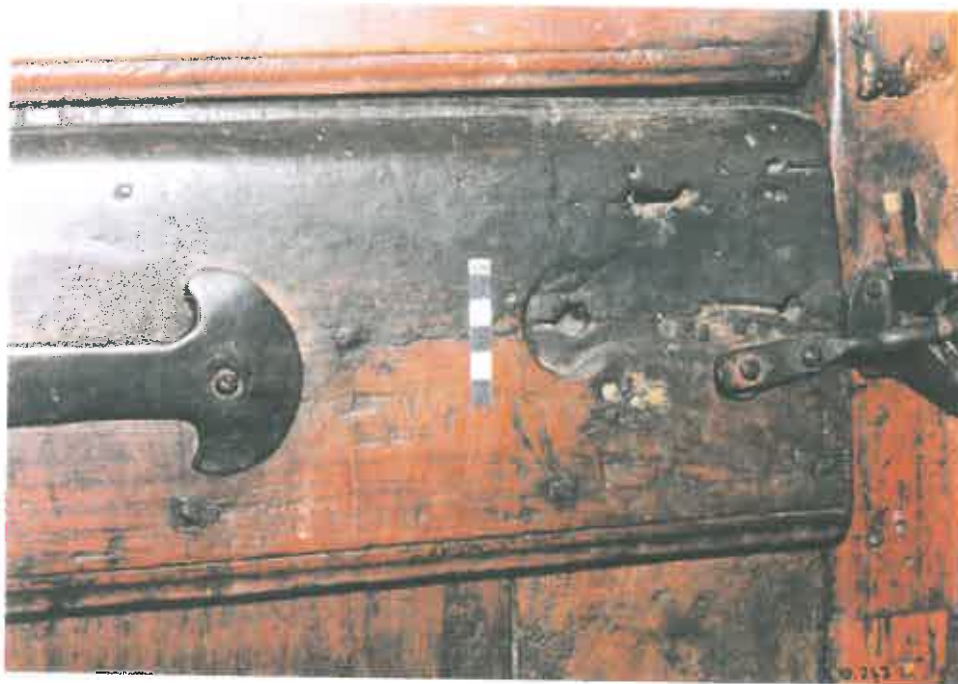
65. A close-up of the late 19 th century latch, with markings of much earlier latches (scale 5cm).
