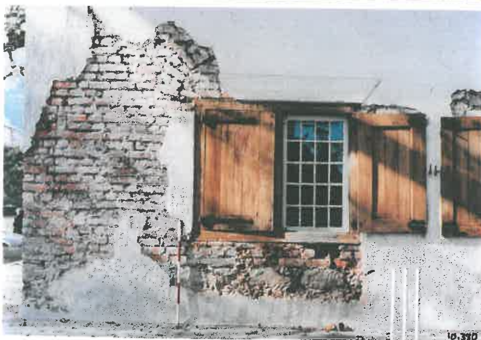
47. On the far left, the relieving arch above the casement is visible. The same type of brick and granite were used as in the front façade (scale 1m)(looking E).
