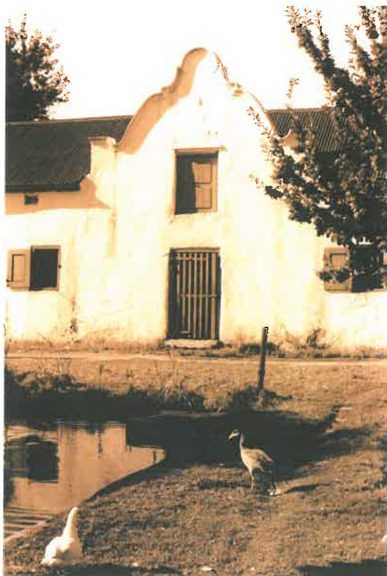
112. An excellent photograph of the wine-cellar, showing the later slatted door, modernised shutters, old tin roof and the tranquility of the old dam (Willem Malherbe 1965, neg. 9).
