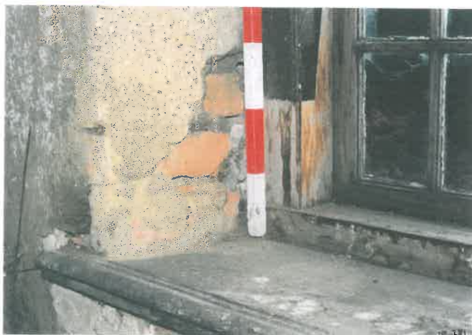
75. The window-sill is exceptional and similar to those used on the interior of the house.
