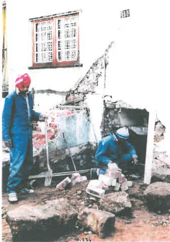
89. In preparation for the study, workers take out some of the huge granite blocks of the old wall.
