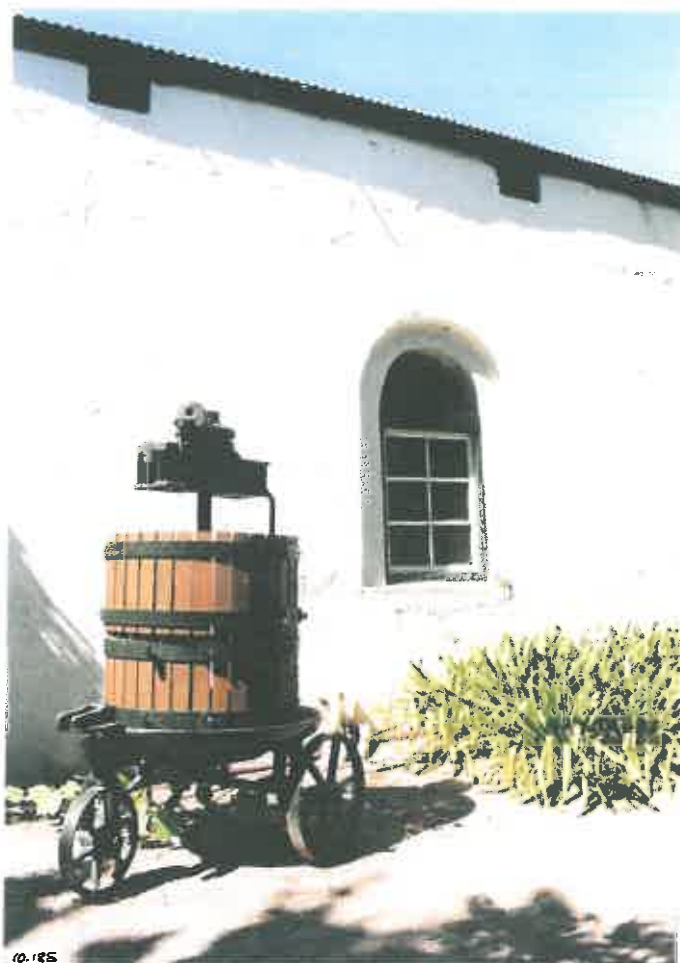
139. On the exterior the old holes for the beams are visible in the plaster work (looking N).
