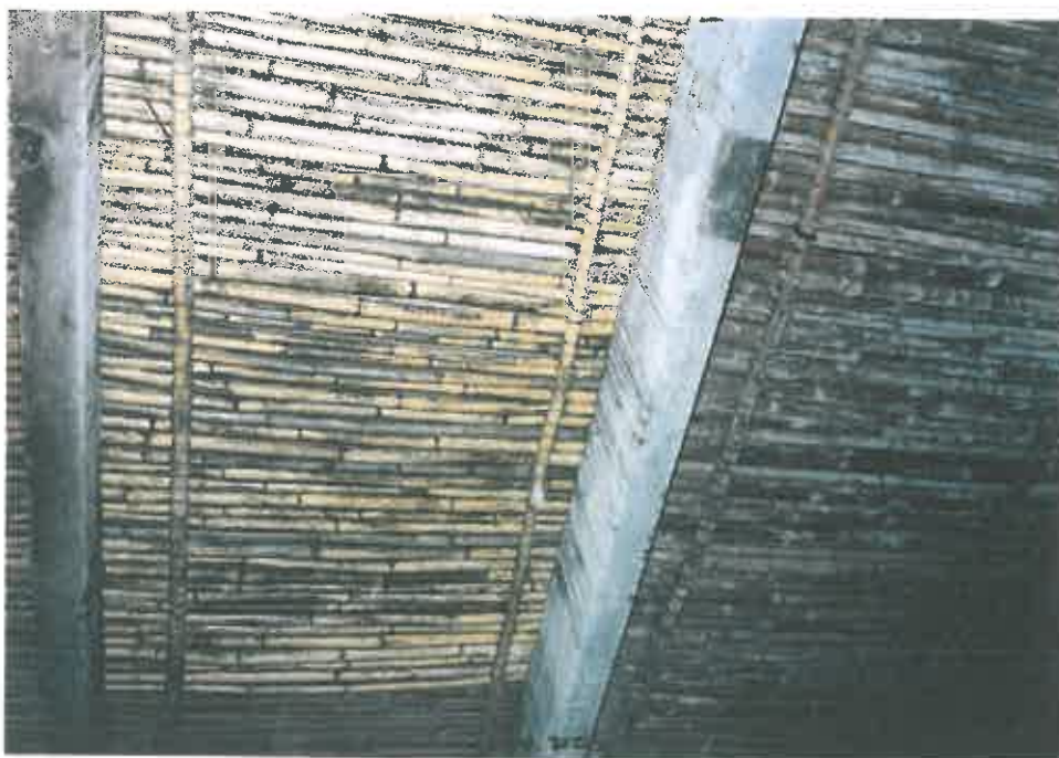
125. Most of the other beams are of the (late) 19 th century, and the yellowish reeds cover an old entrance to the loft.
