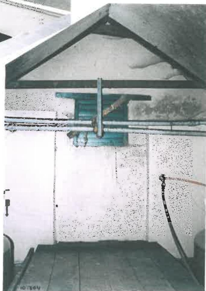
137. A view on the interior of this little window, showing an opening where presumably a door was.
