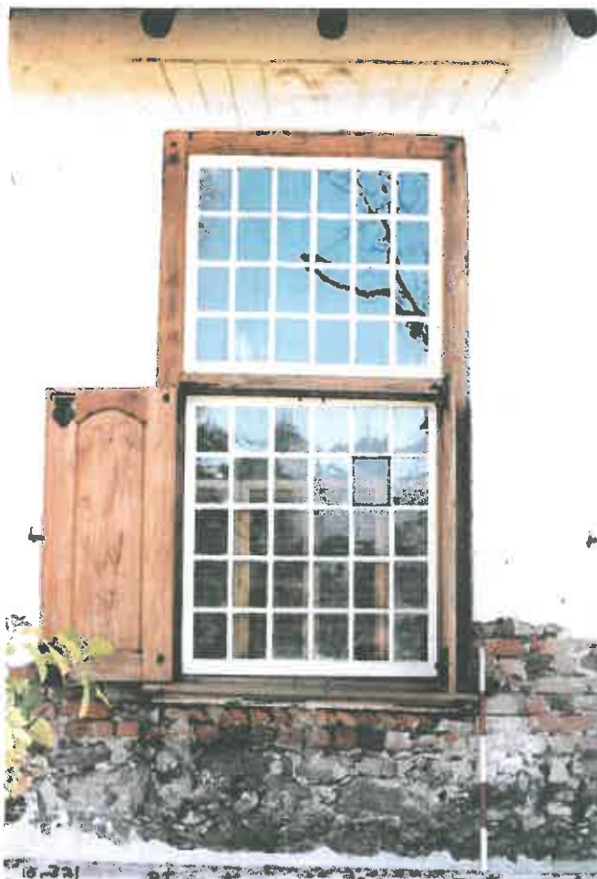
24. Below the sash-windows (Room C) the granite walling with hard-fired brick is obvious (looking W)(scale 1m).
