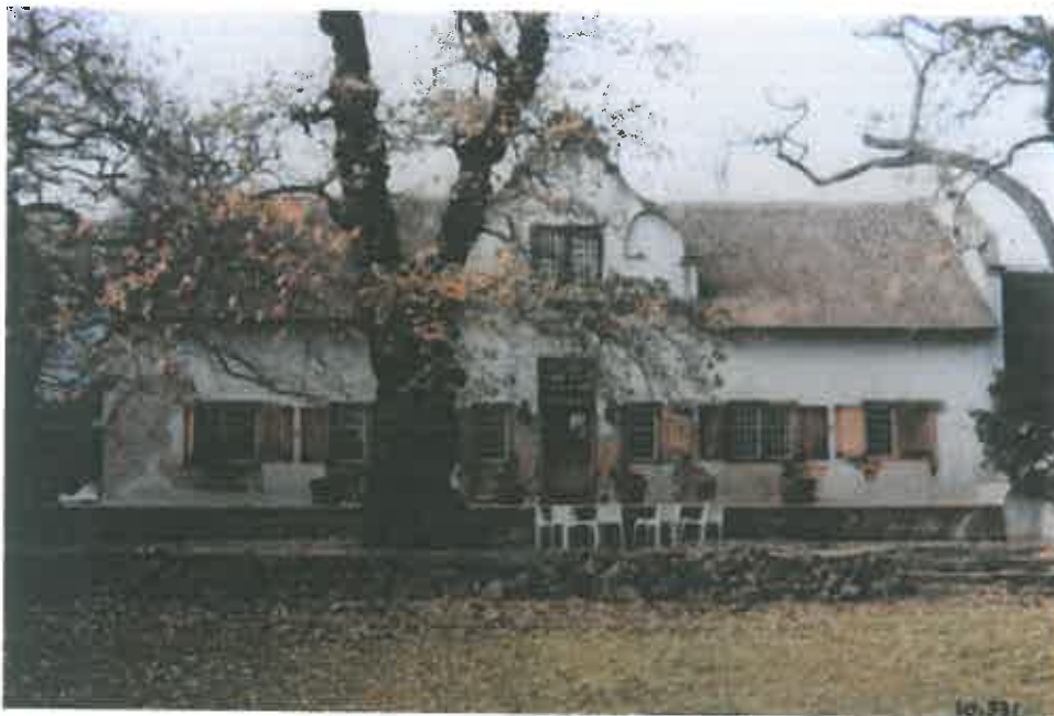
46. A view of the rear with its unpainted casements and shutters during 1979 (GB).
