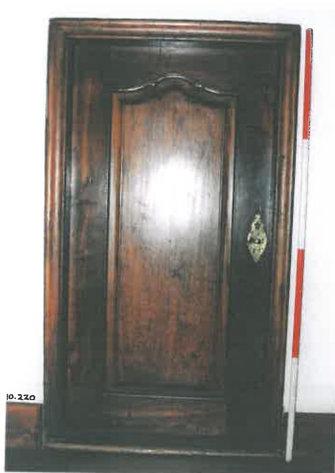
42. There are seven of these gabled doors, which to my mind, could date to the 1770s. They all display signs of older locks and rotary handles, now absent.
