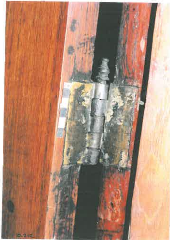
40. One of the front door's cylindrical hinges in brass (scale 50cm).
