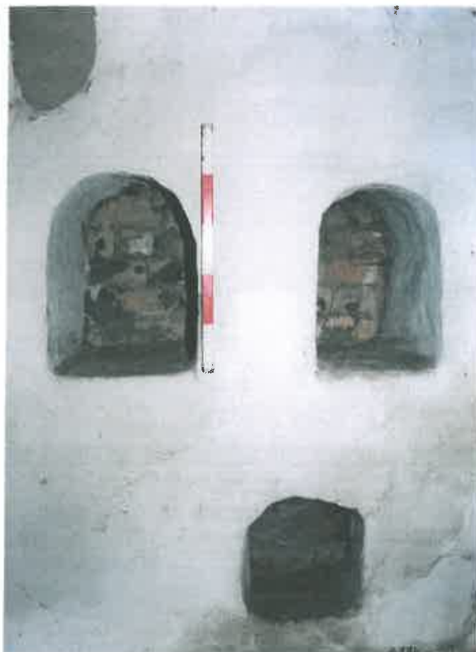
81. The two tiers of nests have been neglected and should be sensitively restored (scale 50cm)(looking N).
