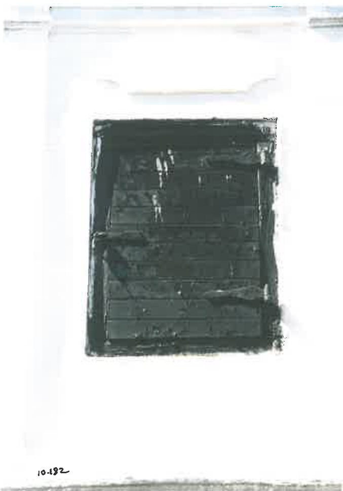
10.132 131. The dormer shutter/door of the central gable may date to early 1900. The casement is older.
