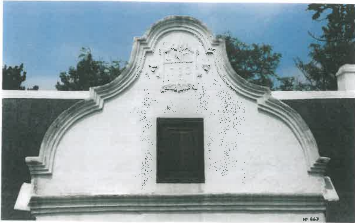
4. This fine holbol gable was erected in 1780 by Dirk Hoffman unto an earlier 18 th century outbuilding. The single casement replaced a double casement.
