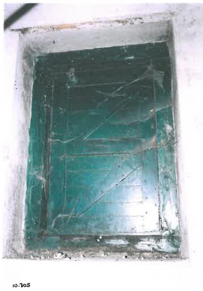
10.1305 132. The interior of the same, with an old lintel.
