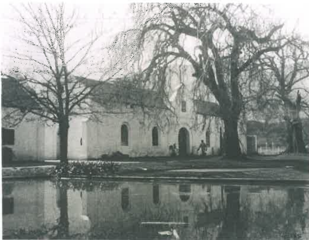
FIG.67 A fine view of the wine-cellar, probably in the 1940s, with the large dam in the foreground. Note the appendage then had square doors (Courtesy GB).
