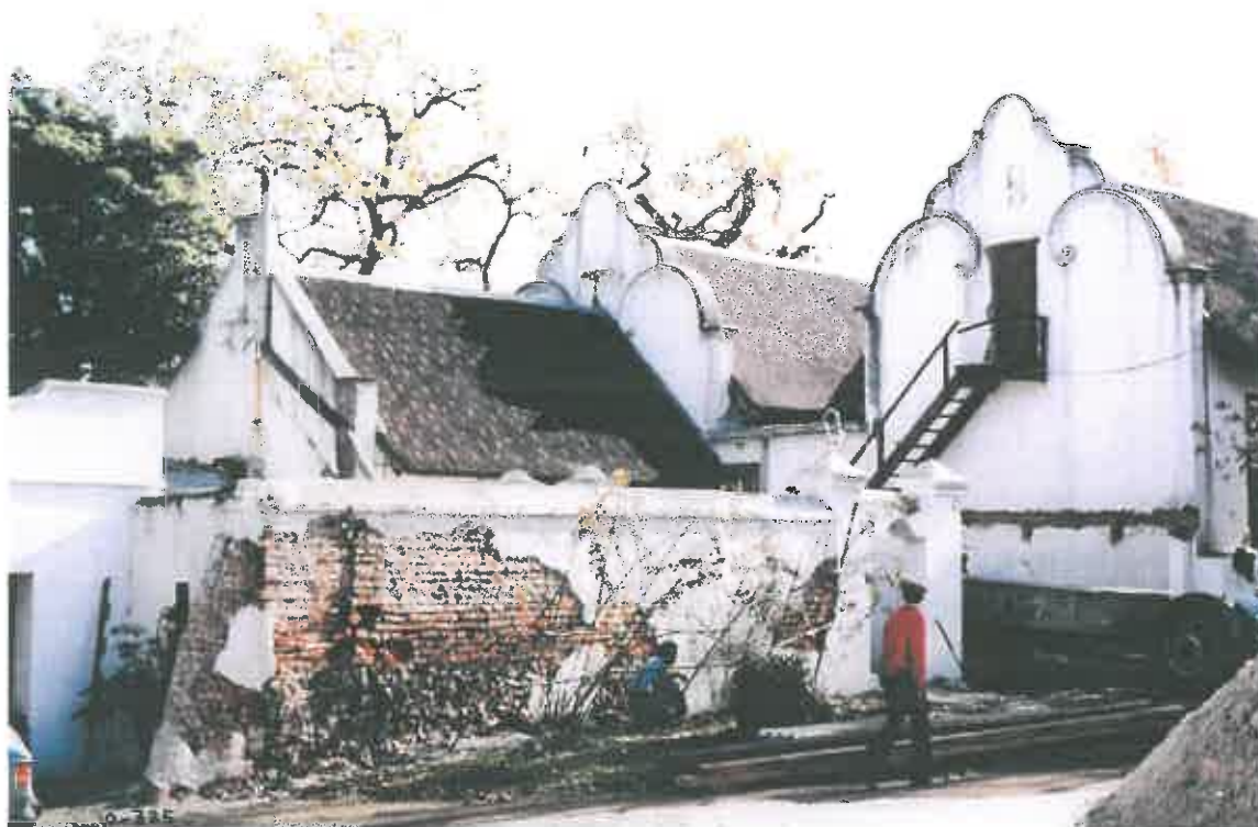
82. In 1979 a portion of the fowl-run wall was exposed, indicating river stones and granite as a base for the upper brickwork. The study was in the process of being constructed.
