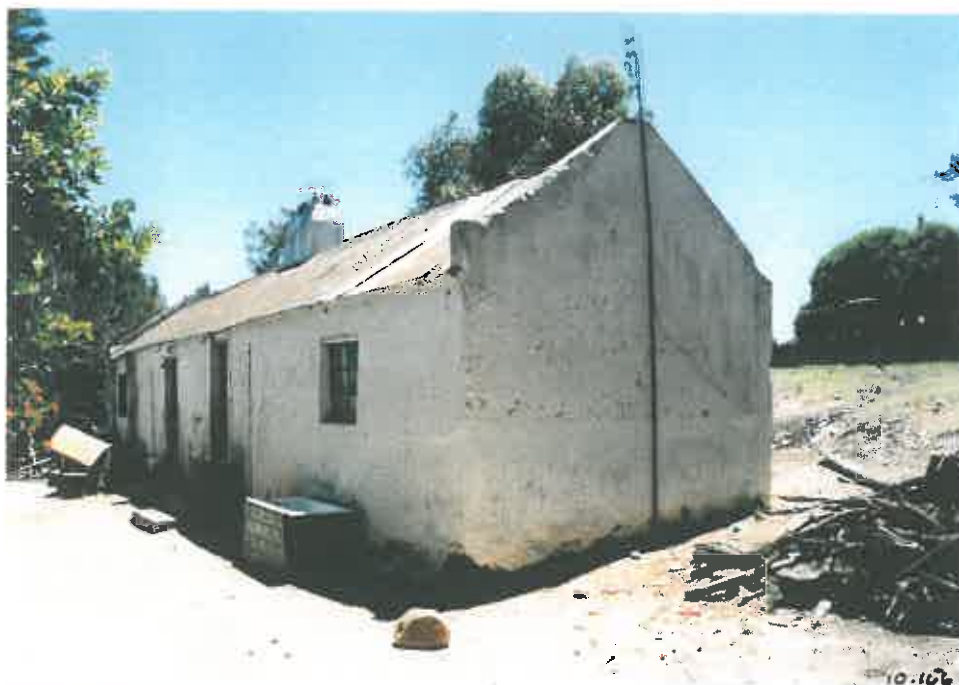
146. The same cottage, from its eastern end (looking W).
