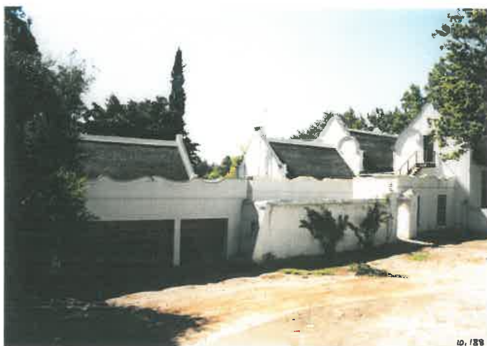
6.3 Note the prominence of the fowl-run, being in line with the façade of the homestead.
