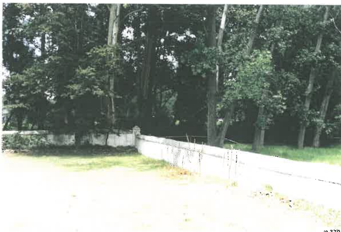
15. The western boundary wall continues south to meet a high wall of similar age (looking S).
