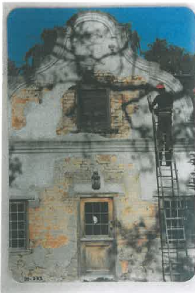
96. A view of the front gable where the transom above the front door has been blocked up on the exterior (>1950)(Courtesy GB).
