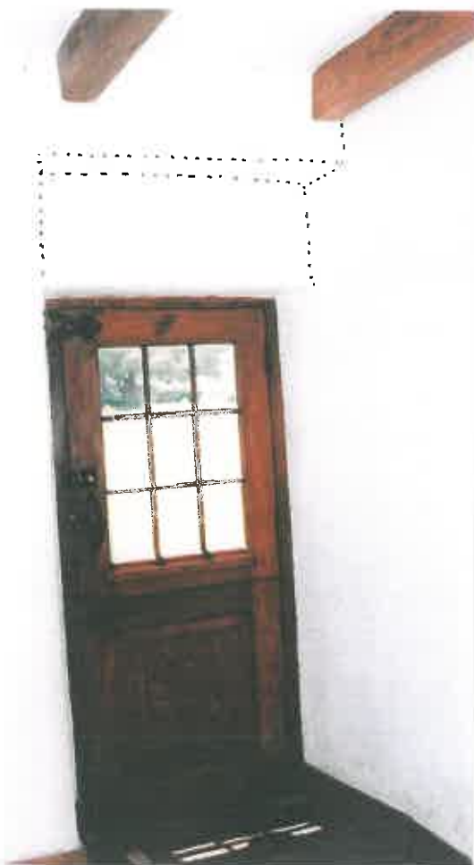
105. In Room C1 the old transom position of the earlier door (see FIG.60) is still visible. The yellowwood beams have been "shaved", but traces of black charring still remain on them.
