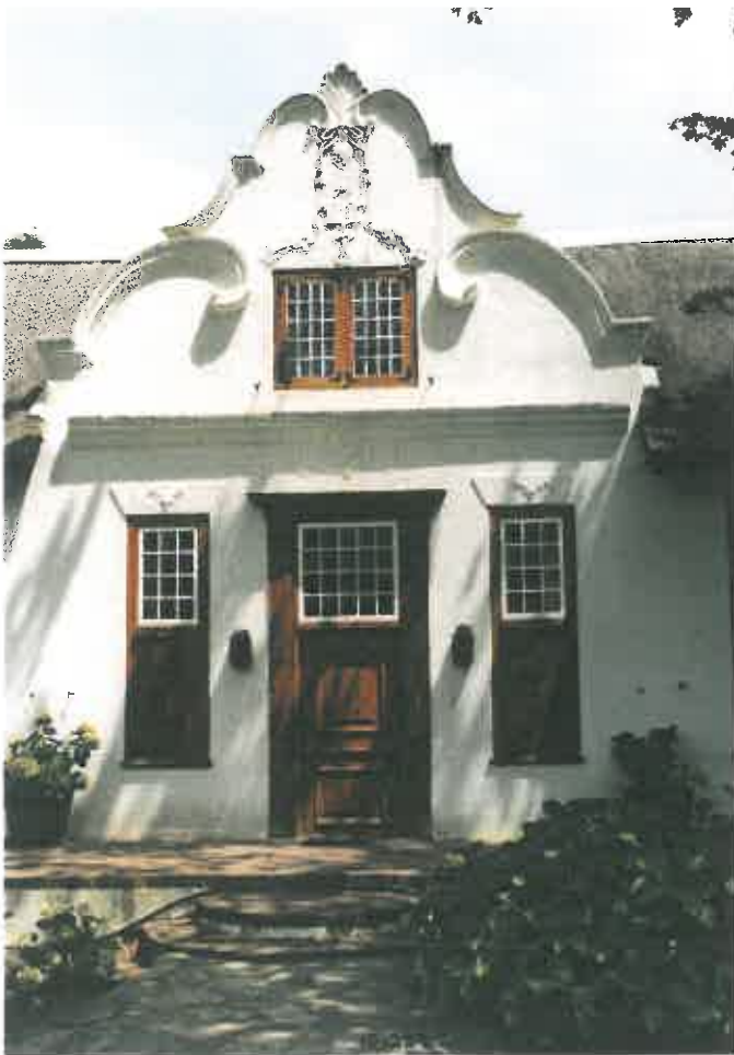
5. The elaborate gables were erected by Dirk Hoffman in 1789. Much is left to the imagination, as the tin roof (c.1890) clipped the gables. Front gable was supplied with later sashes and rear gable with original casements.
