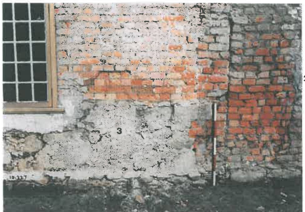
99. West of the right casement was the brick walling for the arch of a coach-door (1), blocked up in brick (2), and the high granite walling (3) as waterproofing.
