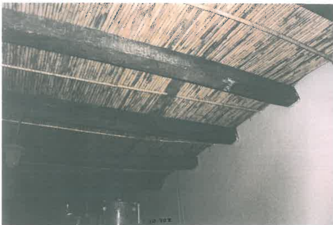
138. At the eastern end of the wine-cellar are a number of old 19 th century beams, very sturdy. The reed ceiling is only loosely packed (looking W).
