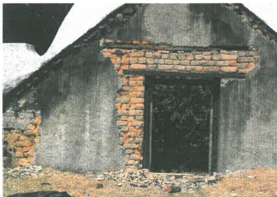
116. The older brickwork of the gable also showed, as well as the old casement opening and lintel.
