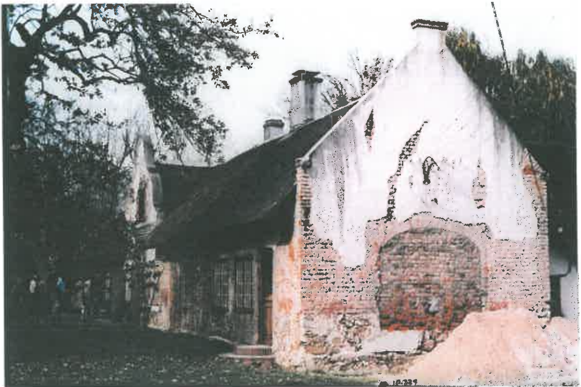
100. A view of the western endgable with the blocked up coach-doors in June 1979.
