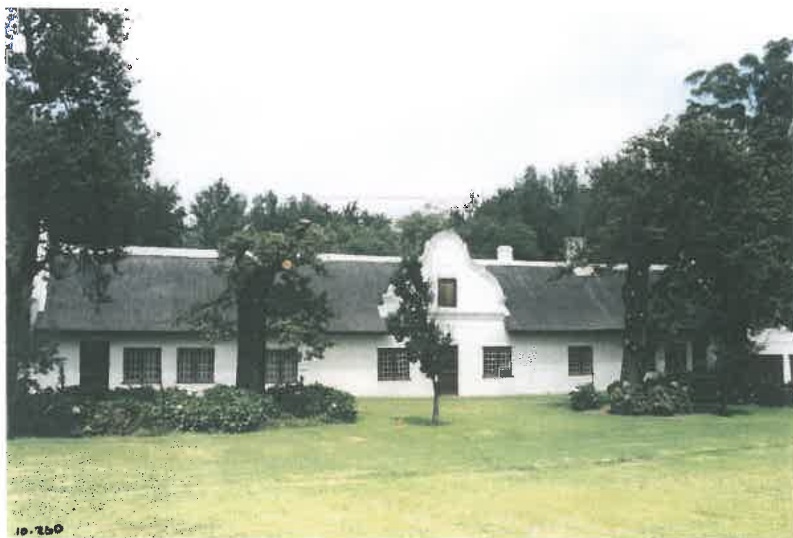
94. A view of the façade of the Jonkershuis, with its >1950 alterations. Note that the thatch comes too low and that there are too many casements, which should be supplied with shutters.
