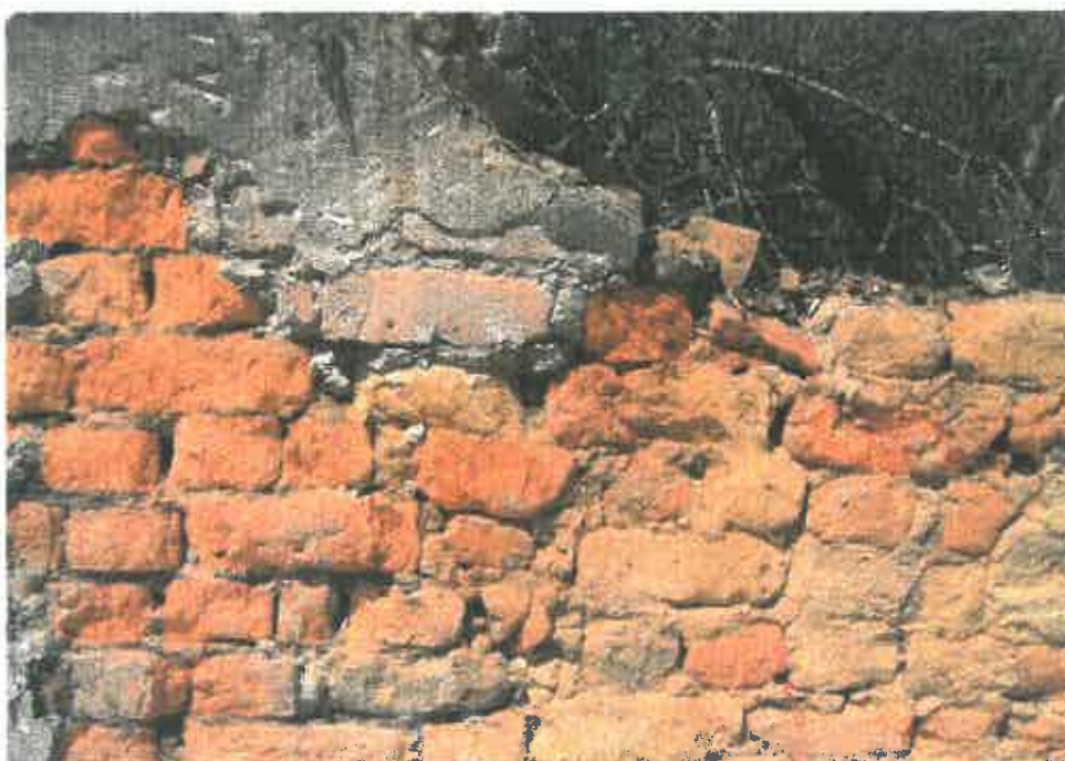
120. Detail where the two periods (18 th and 19 th century) meet (both by Johan Malherbe 2001)(looking S).
