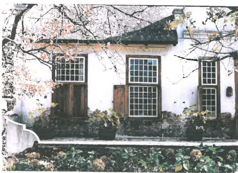
25. A view of the sash-windows (upper part fixed), with their clear panes. Below this part of the stoep, on the soil, author picked up greenish-tinted window glass of the 18 th century.
