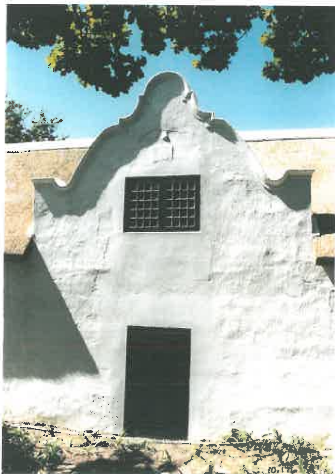
114. The old plasterwork with its rough finish has been retained, and the old casement placed horizontally. The outline of the "c.1800" gable dates to after 1950. Cobbling below the dripline of the thatch is recommended for this building.
