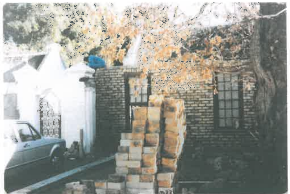
90. The erection of the study under way (courtesy GB, 1979).
