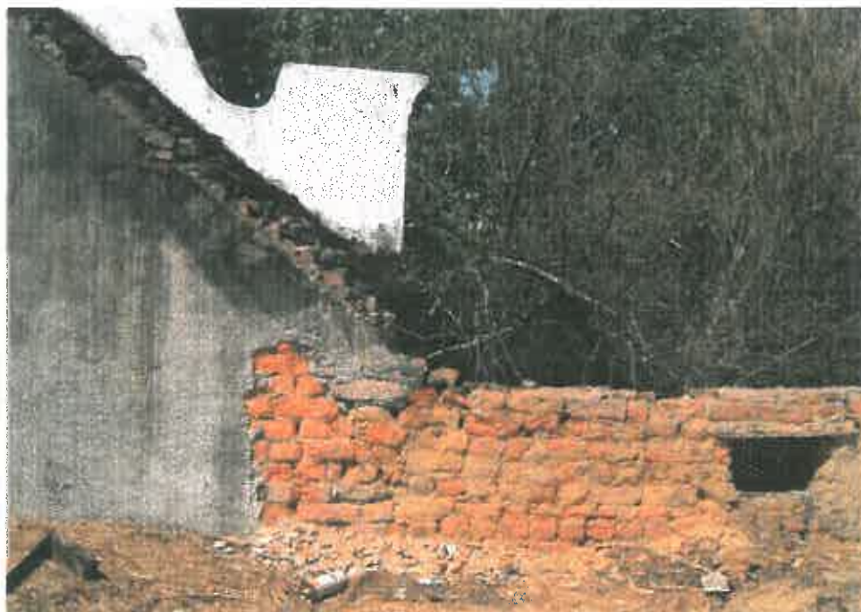
119. On the interior of the gable, the c.1890 brickwork in yellow mortars abuts the older gable with its orange brickwork in grey mortars.
