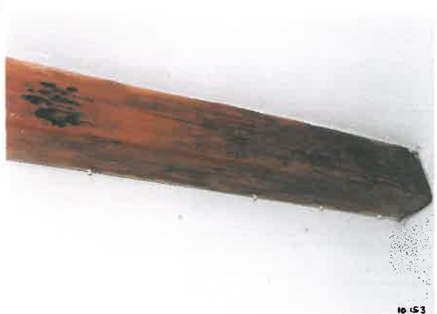
105. In Room C1 the old transom position of the earlier door (see FIG.60) is still visible. The yellowwood beams have been "shaved", but traces of black charring still remain on them.
