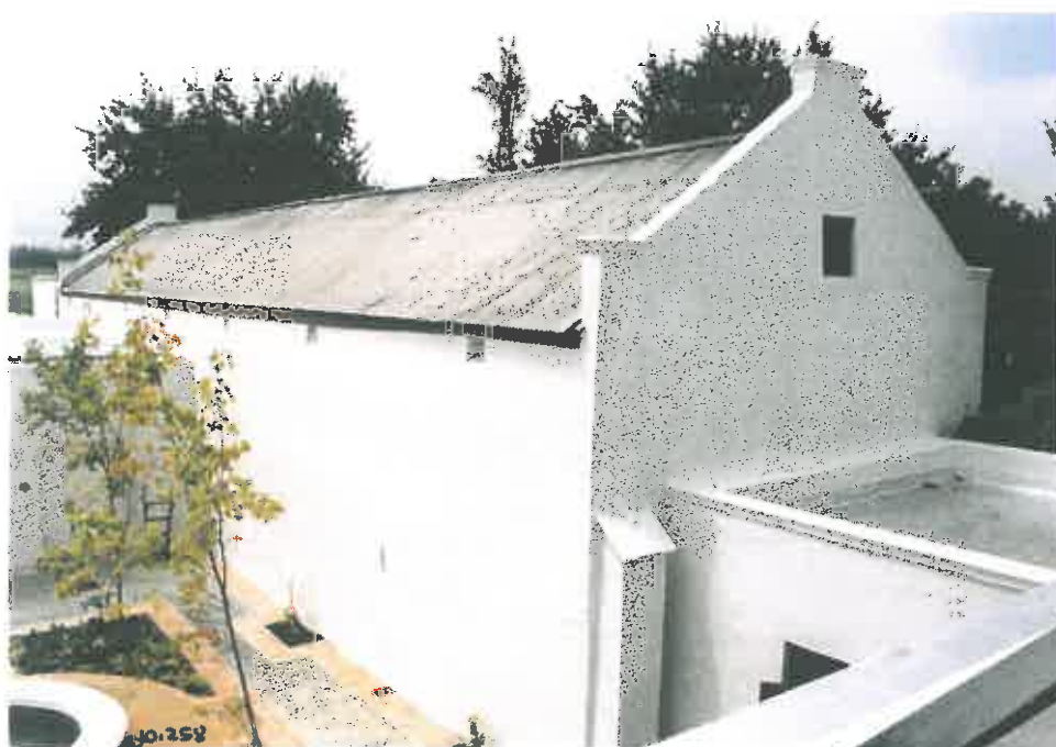
136. View of the rear of the building with at least three ventilation shafts. They were once longer. Note that the end-gable "chimney" is incorrect for this period. The little window is placed in an older opening.
